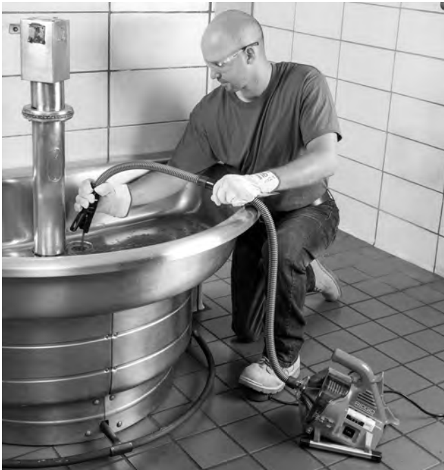
Figure 11 – Retrieving Cable
